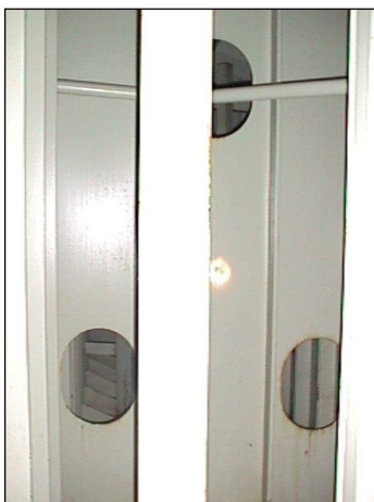
Figure 13: Existing Stability Tank Central Partition and Openings
